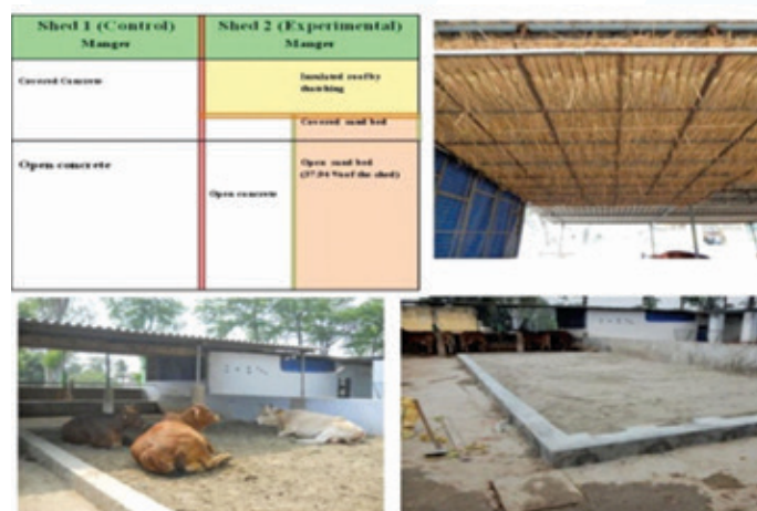
Roof ceiling thermo-protection by paddy straw and floor comfort by sand bed in cow shed
