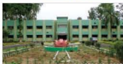
Main Building of ERS, Kalyani
